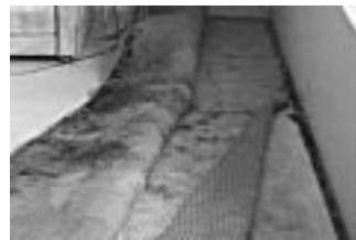
Mold in carpet system caused by vapor emission from slab.
