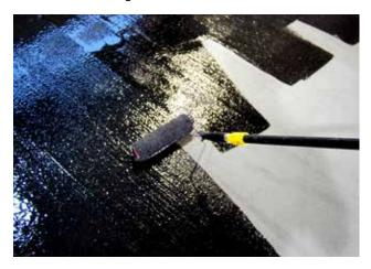
When moisture emission levels exceed the maximum allowed by the wood flooring manufacturer, moisture-mitigation systems are necessary. This one-coat, epoxy resin rapid-set moisture control system can be ready to prime as soon as four hours after it is applied.
