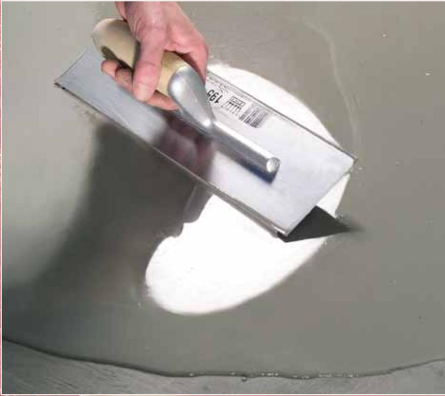
Sub-floor smoothing compounds, or underlayments, are cement-based materials that are generally fluid during application. They set and harden to form a hard, absorbent, smooth surface suitable to receive floorcoverings. They can be used to smooth out imperfections in a sub-floor which would otherwise be mirrored through the final floor finish. They may also be used as a
